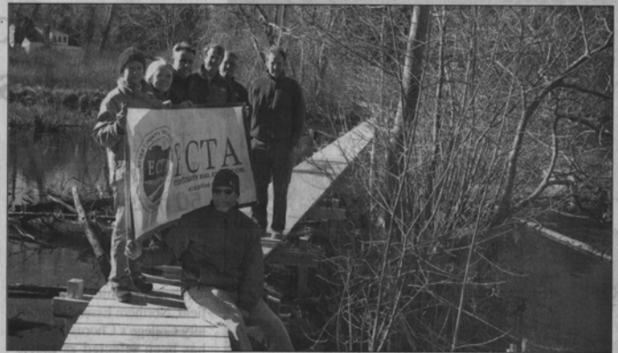
Volunteers show off the newly finished boardwalk at Willowdale State Forest.
